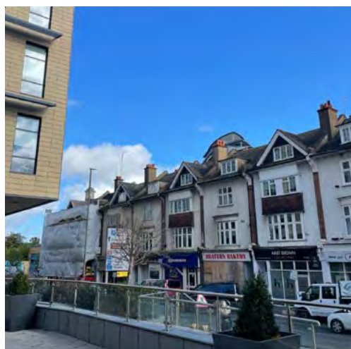
Fig. 40: Site photograph of 2-7 Guildford Road
