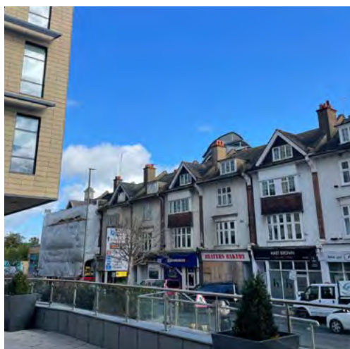
Fig. 35: Site photograph of 2-7 Guildford Road
