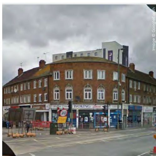
Fig. 121: Street View image of Victoria House
