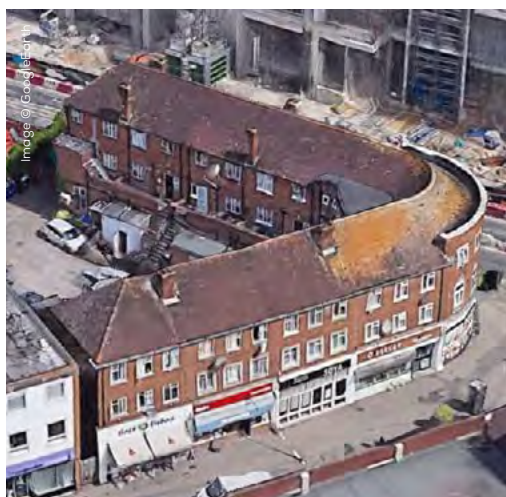
Fig. 120: Aerial image of Victoria House
