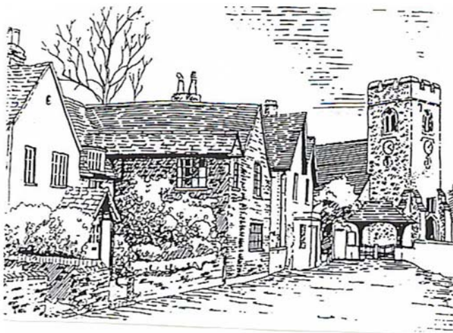
Figure 24: Listed Buildings in Church Street (extract from Conservation Area Appraisal)
