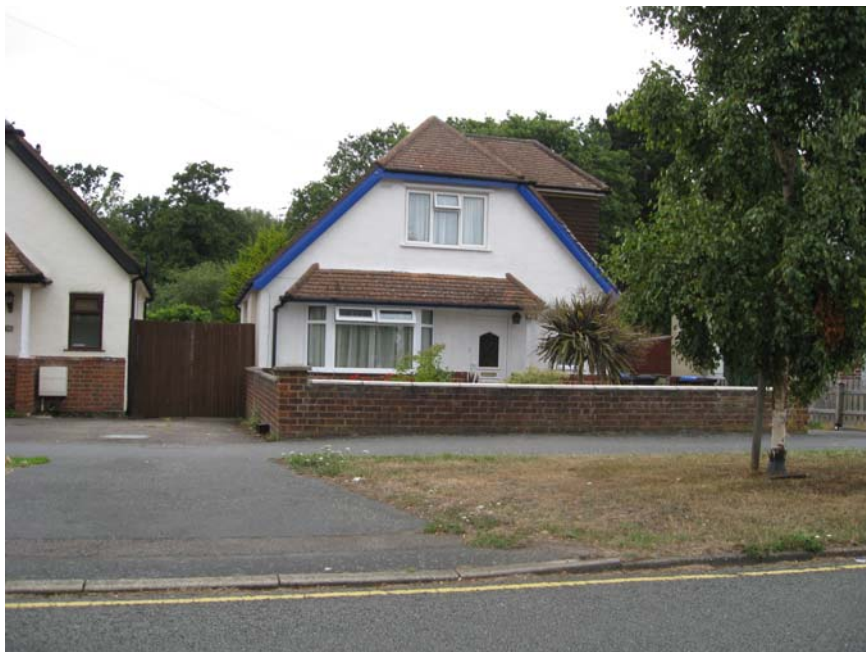
Figure 31: House on Woodlands Avenue with asymmetric roof, painted render and coloured fascias
