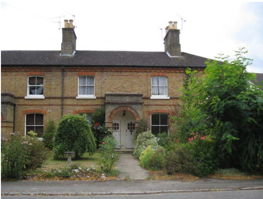
Figure 13: Retained properties on Wellington Terrace
