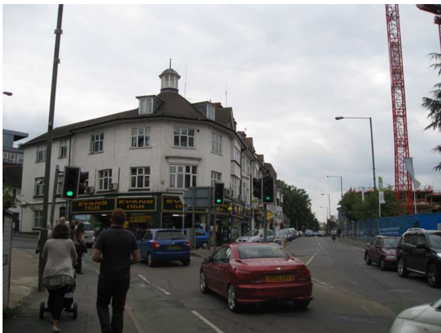
Figure 19: Victorian buildings and new development on Guildford Road
