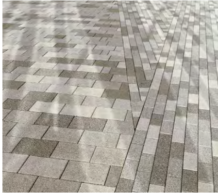
Granite style paving to main entrance, central boulevard and pedestrian boundary route
