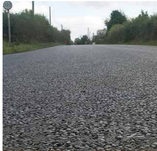
Asphalt to carriageway
