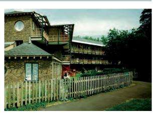
*Figure 24:* In this housing association scheme, solar shading is provided by balconies and overhangs
