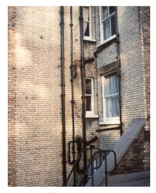
*Figure 9:* White walls require regular maintenance or their reflectance will deteriorate, as shown here
