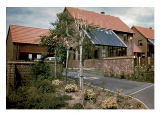
*Figure 32:* At Willow Park, Chorley, careful road layout design means that all the passive solar homes can have a southerly orientation
