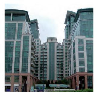
*Figure 7:* A tunnel effect can occur if a window has projecting wings on both sides of it. In this development in South London (architects Broadway Malyan), the windows have been increased in size to compensate.
