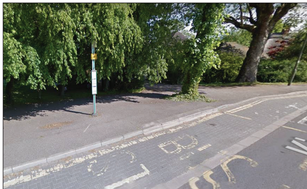
Figure 5.9 – Eastbound Bus Stop on Kingfield Road
