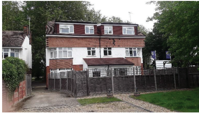
Photograph 1 View of Building B10, with low potential to support roosting bats, viewed from the south.
