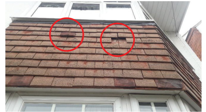
Photograph 5 View of lifted hanging tile and missing tile under window on building B11, on southern elevation.
