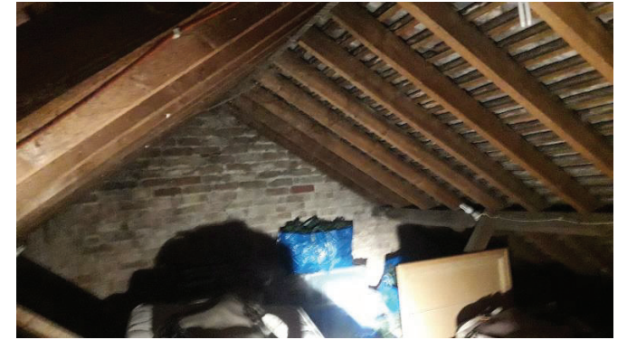
Photograph 6 View of inside of loft void of B11, with unlined tiles.
