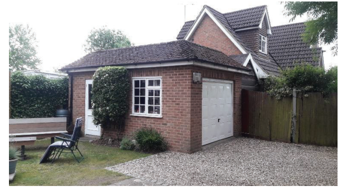
Photograph 7 View of garage building B11c, as viewed from the north-west, with negligible potential to support roosting bats.
