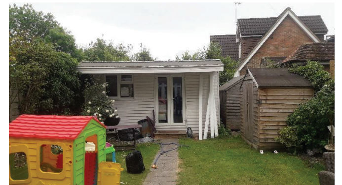
Photograph 8 View of sheds and outbuilding B11d, as viewed from the north-west, with negligible potential to support roosting bats.
