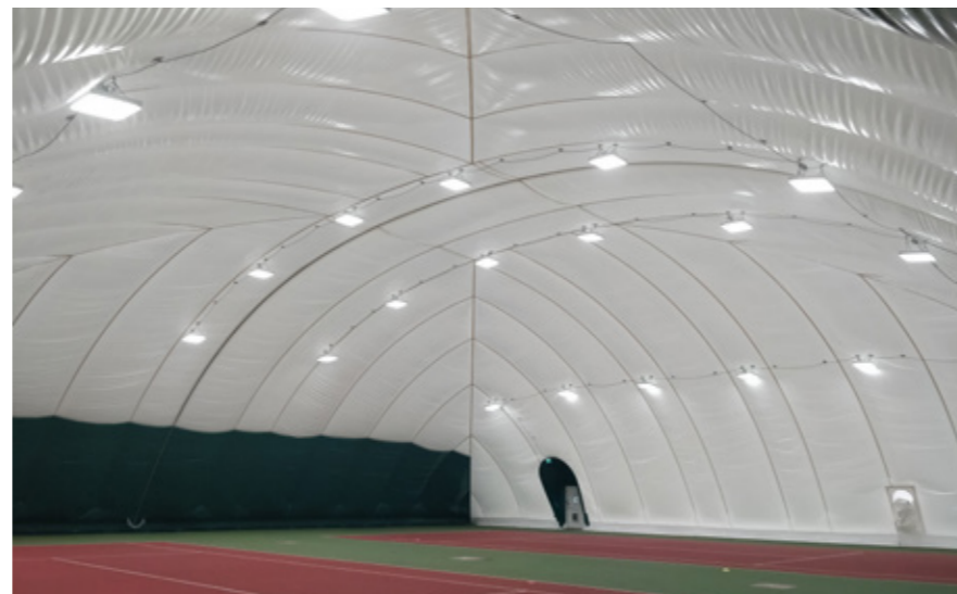
INTERNAL OF TYPICAL AIRDOME
