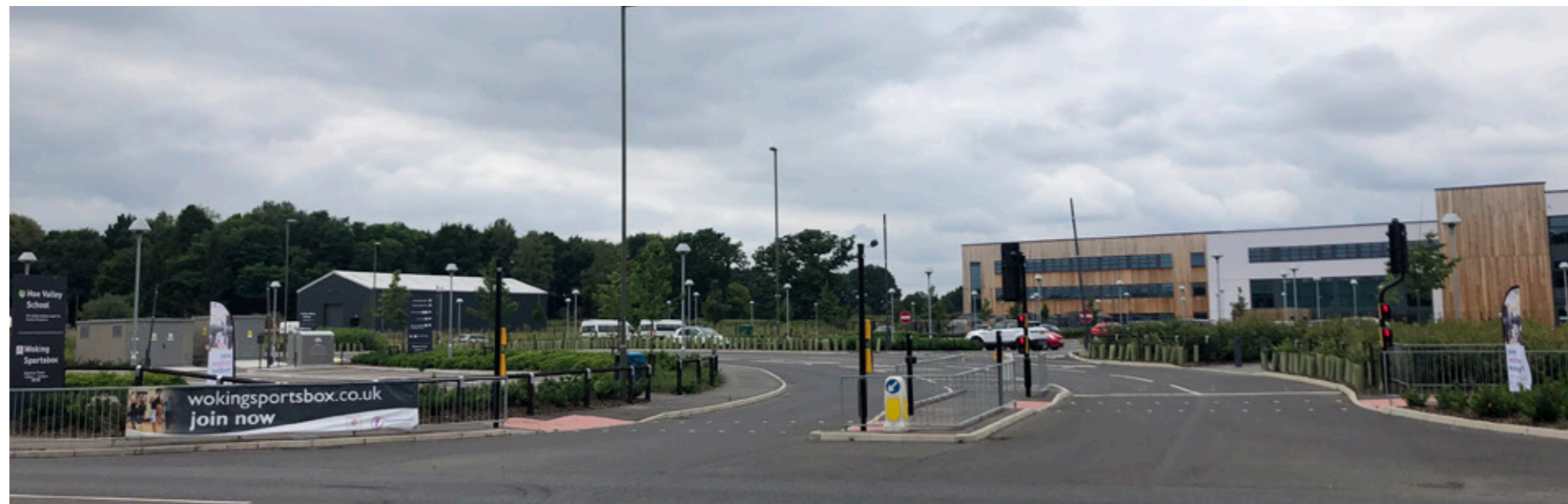
PHOTOGRAPH 3 - SITE ENTRANCE FROM EGLEY ROAD
