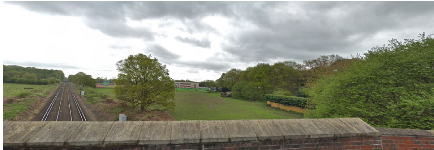
PHOTOGRAPH 1 - VIEW FROM WEST OVER RAILWAY BRIDGE
