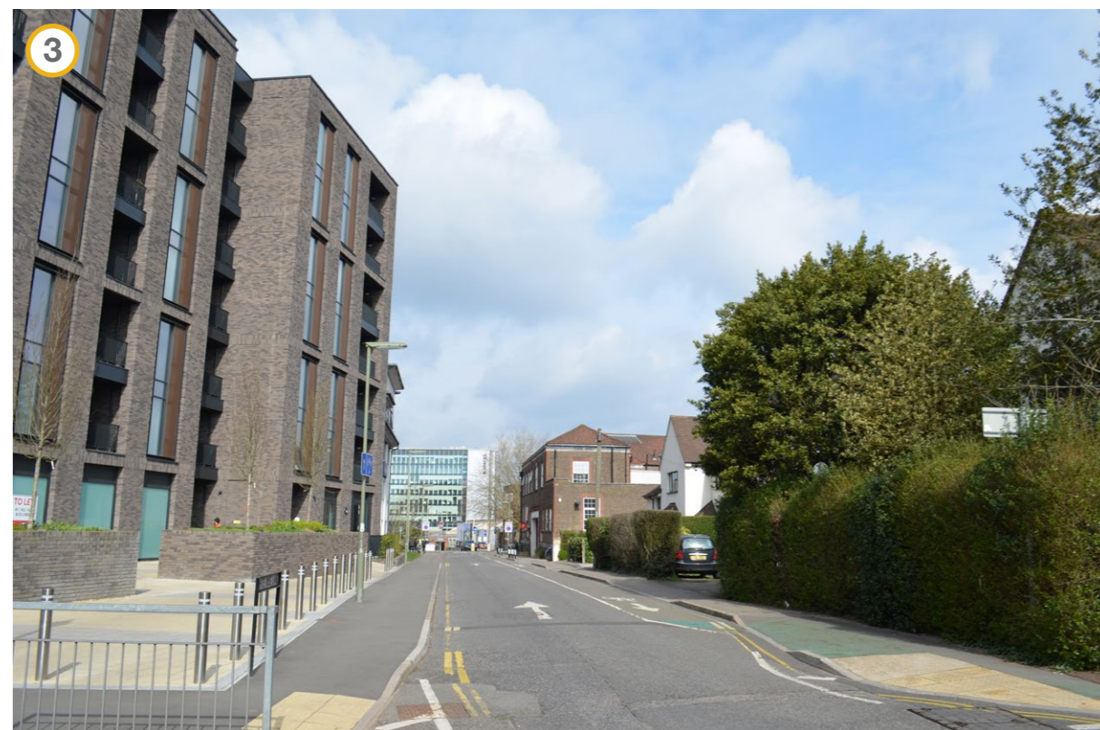
FIGURE 5 : Image 3 showing newly constructed Harrington Place looking North
