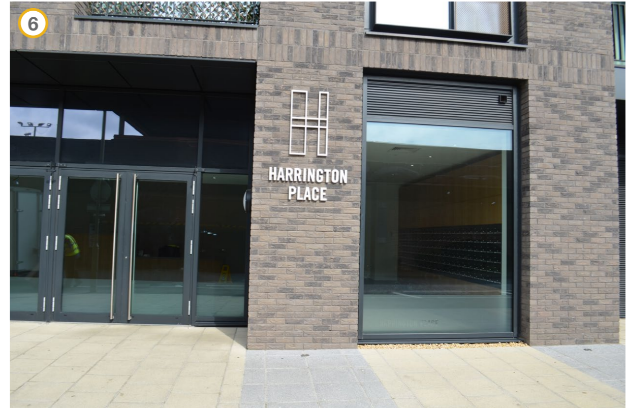
FIGURE 8 : Image 6 showing newly constructed Harrington Place looking at entrance
