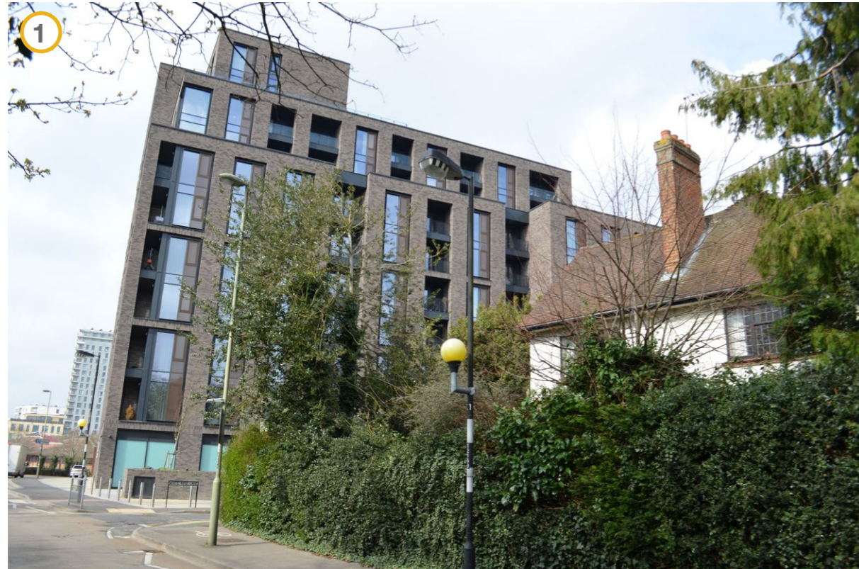
FIGURE 3 : Image 1 showing newly constructed Harrington Place approaching from East
