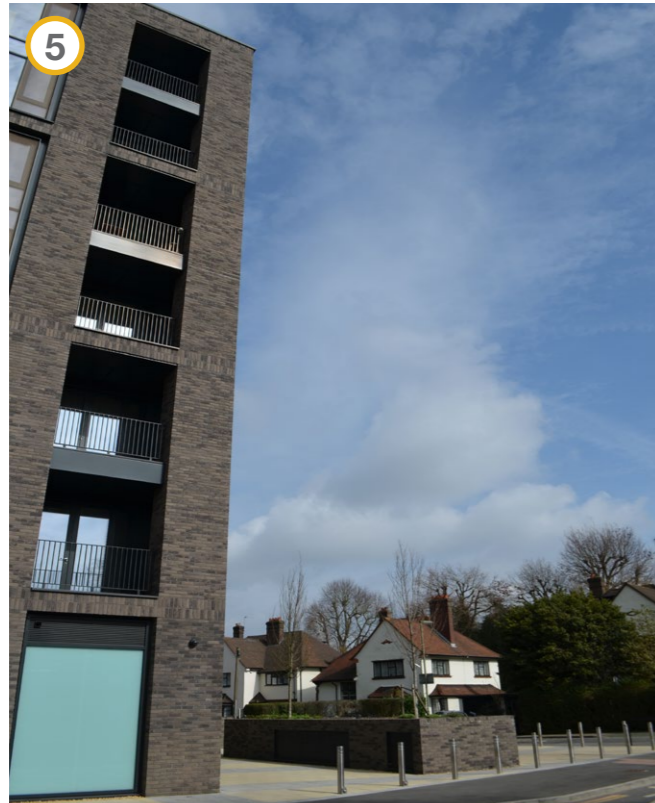
FIGURE 7 : Image 5 showing newly constructed Harrington Place looking West
