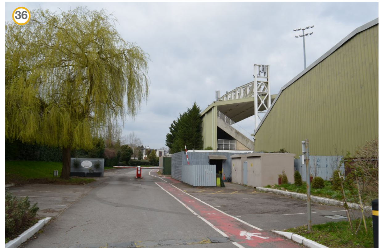
FIGURE 39 : Image 36 view from Site Road behind South Stand looking North West
