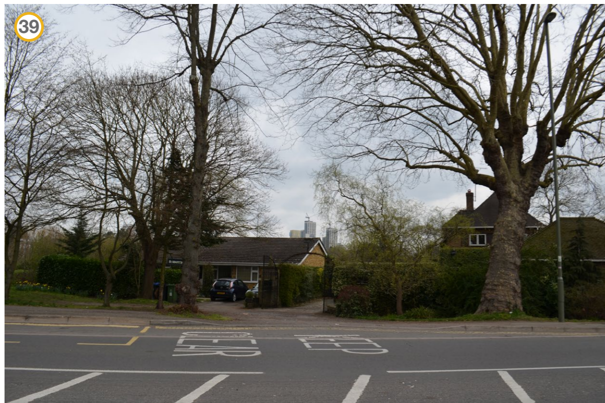
FIGURE 42 : Image 39 view from Kingfield Road looking North towards Woking Town Centre
