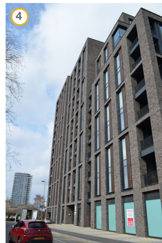
FIGURE 6 : Image 4 showing newly constructed Harrington Place looking East
