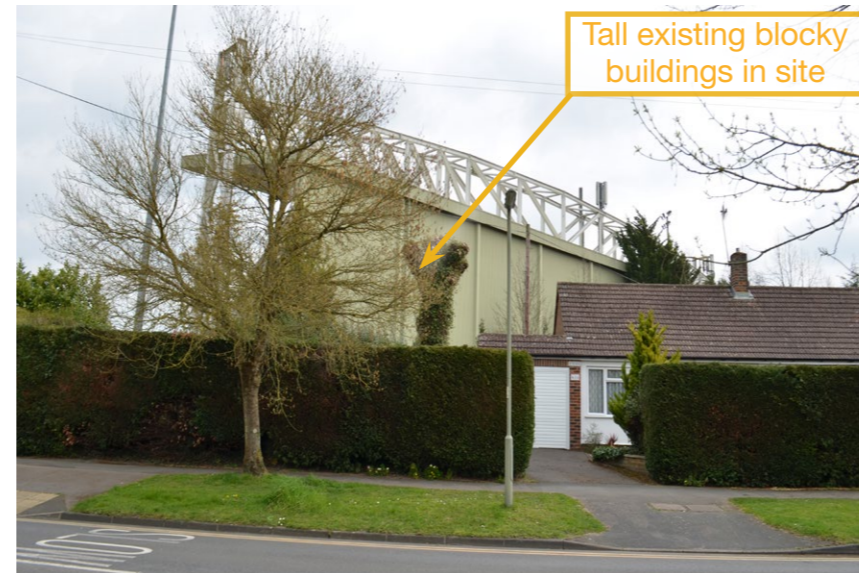
FIGURE 9: View of South Stand from Westfield Avenue
