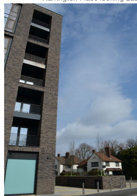
FIGURE 40: Newly constructed Harrington Place looking West
