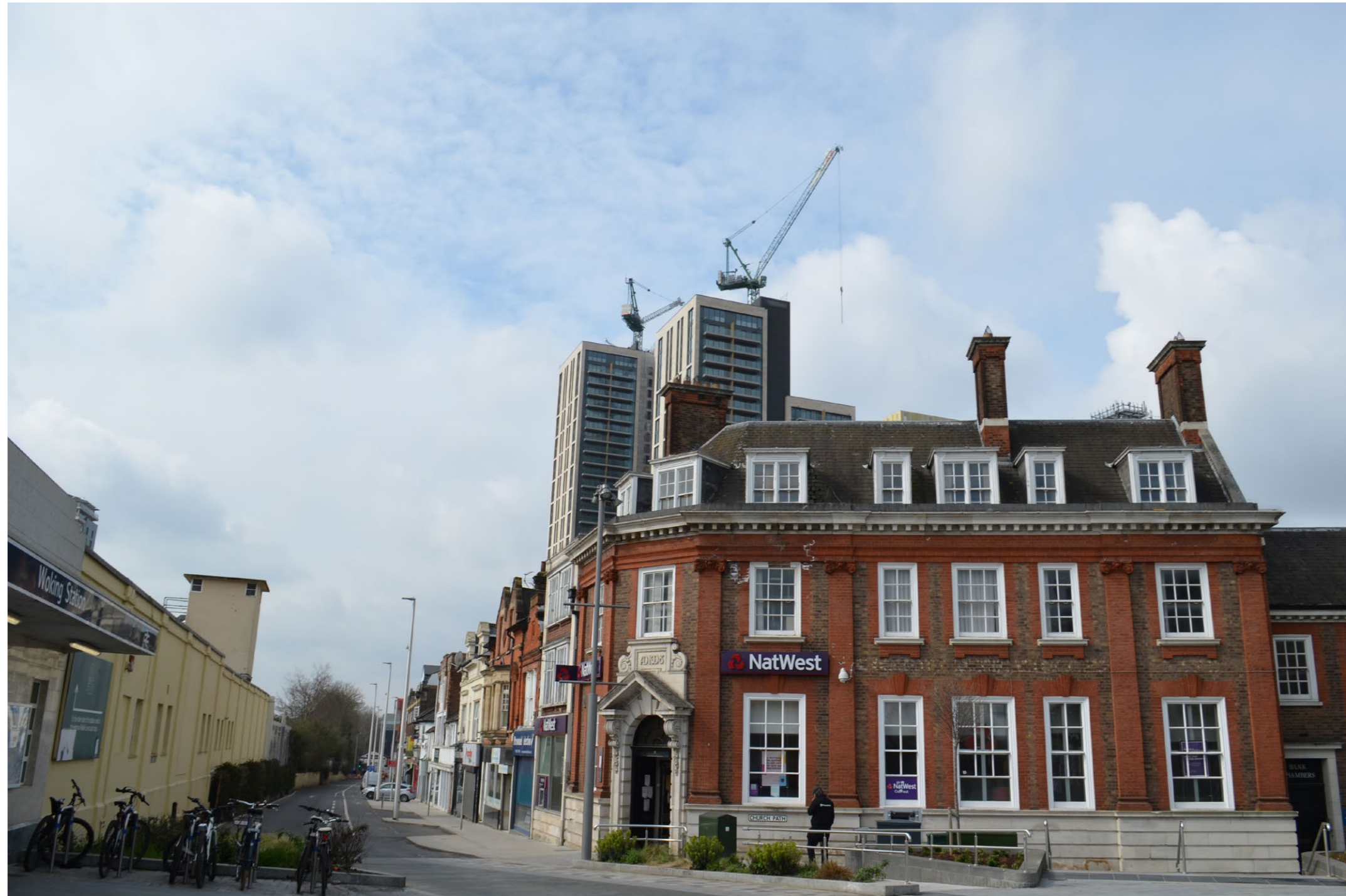
FIGURE 36: Looking from Woking Station on High Street
