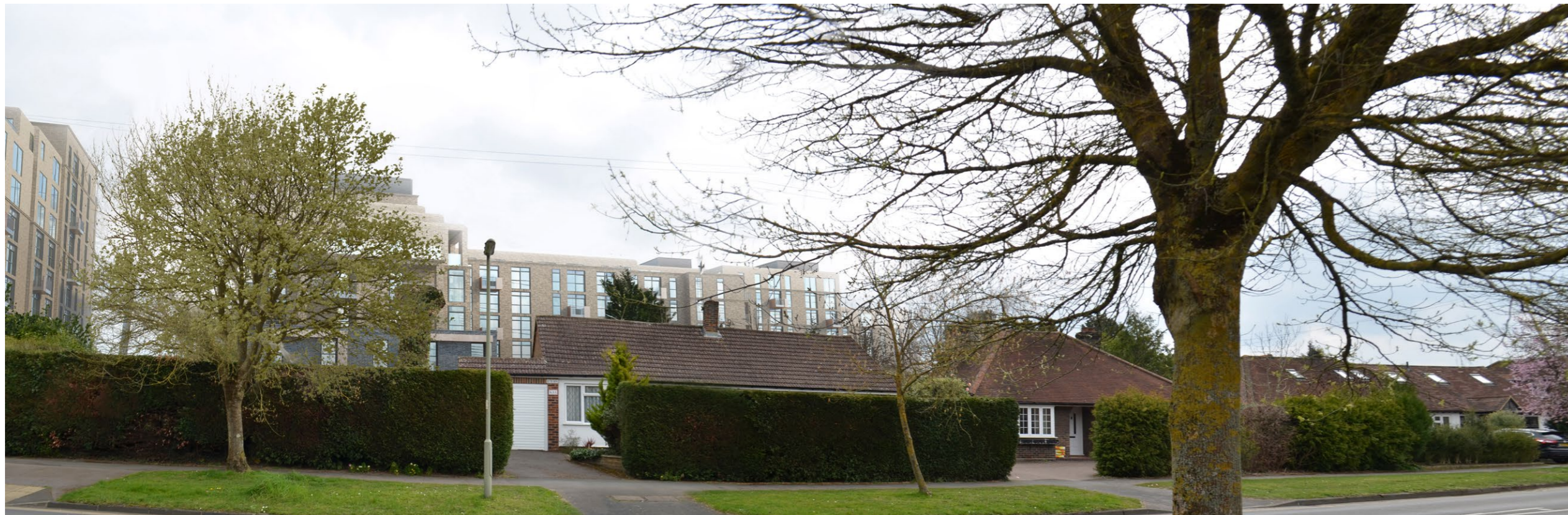
FIGURE 109: Proposed view looking East towards Site next to South Stand behind bungalows along Westfield Avenue (Development 70m from Westfield Avenue)
