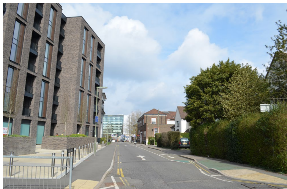
FIGURE 39: Newly constructed Harrington Place looking North
