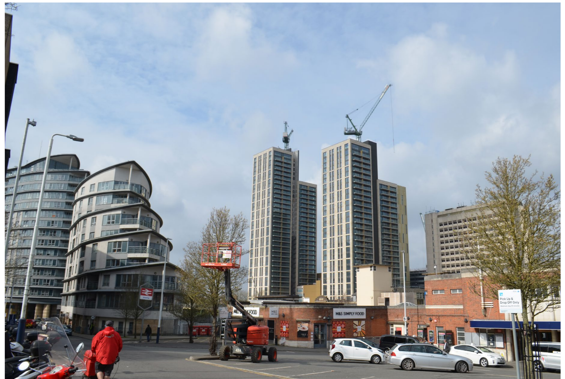
FIGURE 35: Looking towards Woking Station from Station Approach
