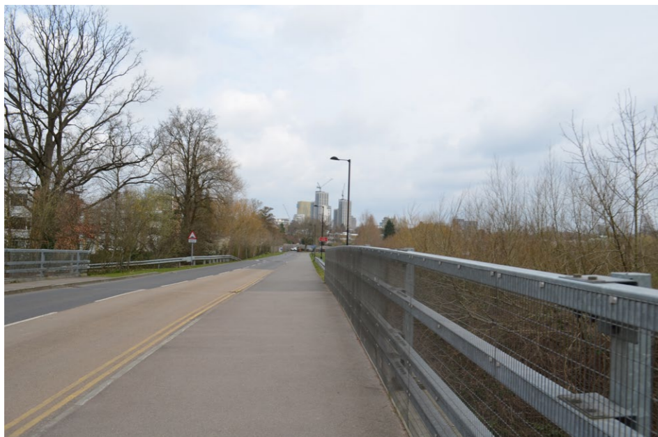
FIGURE 33: View from Hoe Stream looking North towards the Town Centre
