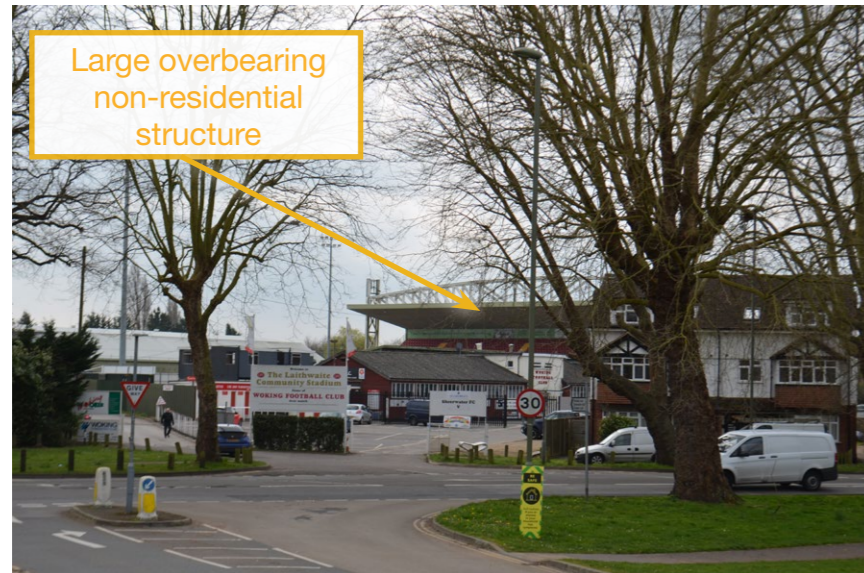
FIGURE 8: View of entrance to the site coming from Woking Park, looking South
